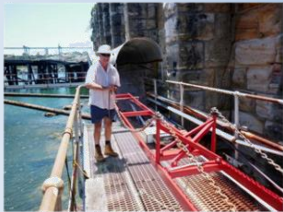
Peter installing chains
