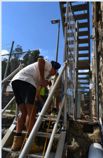
Peter welding the post
