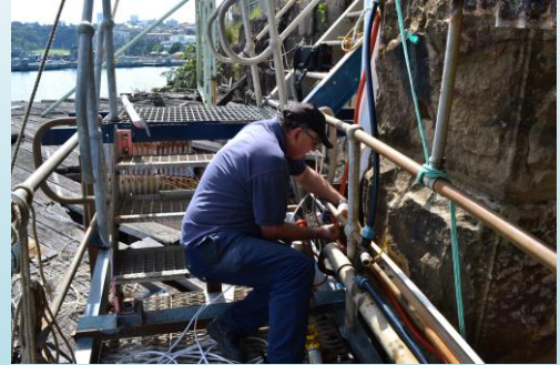
Paul working on the power feed
